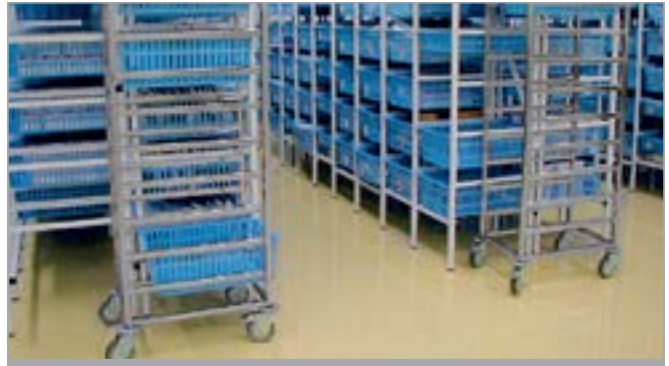
Planning for central storerooms
